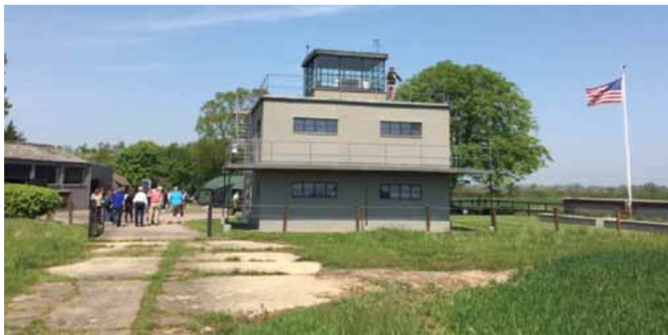
The original 100th Bomb Group control tower at Thorpe Abbots.
