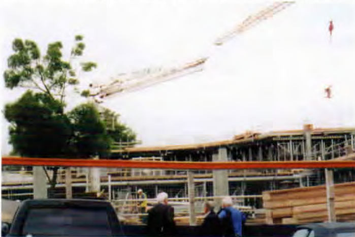
Overlooking the construction
