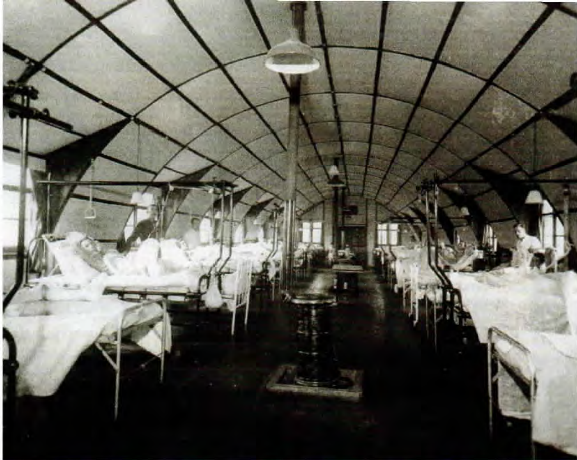
One of several orthopedic wards at 65th General Hospital. Note the small coke stove in foreground, the only source of heat. Ward floors were asphalt, kept waxed.
