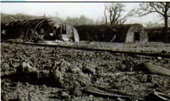
Destroyed and damaged surgical wards at 121st Station Hospital, Braintree, Essex after bombing by the Luftwaffe April 19, 1944.
