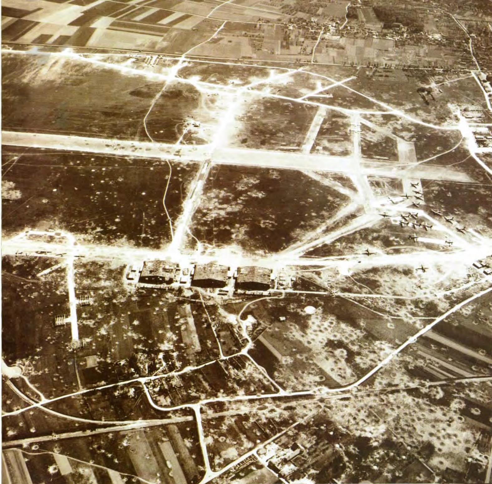
German airfield bomb damage
