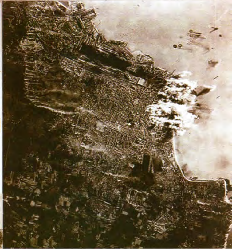
Smoke pots at left of photo - apparently ineffective
