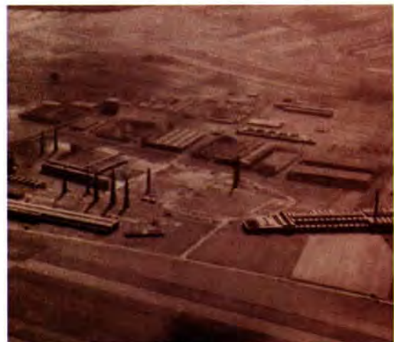
Fake Skoda works looked real at a distance. When attacks started, fires were lit to fool later formations of bombers.
