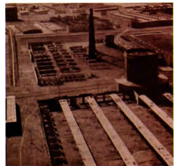
Close view reveals nothing but rectangles of cheap board and canvas "flats" with windows cut in or painted on them.
