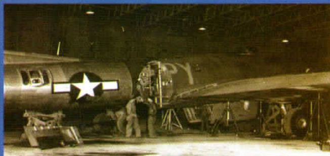
2nd S.A.D. Rear fuselage change STA 547, 5-27-1944, Ser. 42-31828
