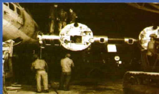
2nd S.A.D. Inner wing panel change "Patches" STA 547, 5-27-1944, Ser. 42-39800
