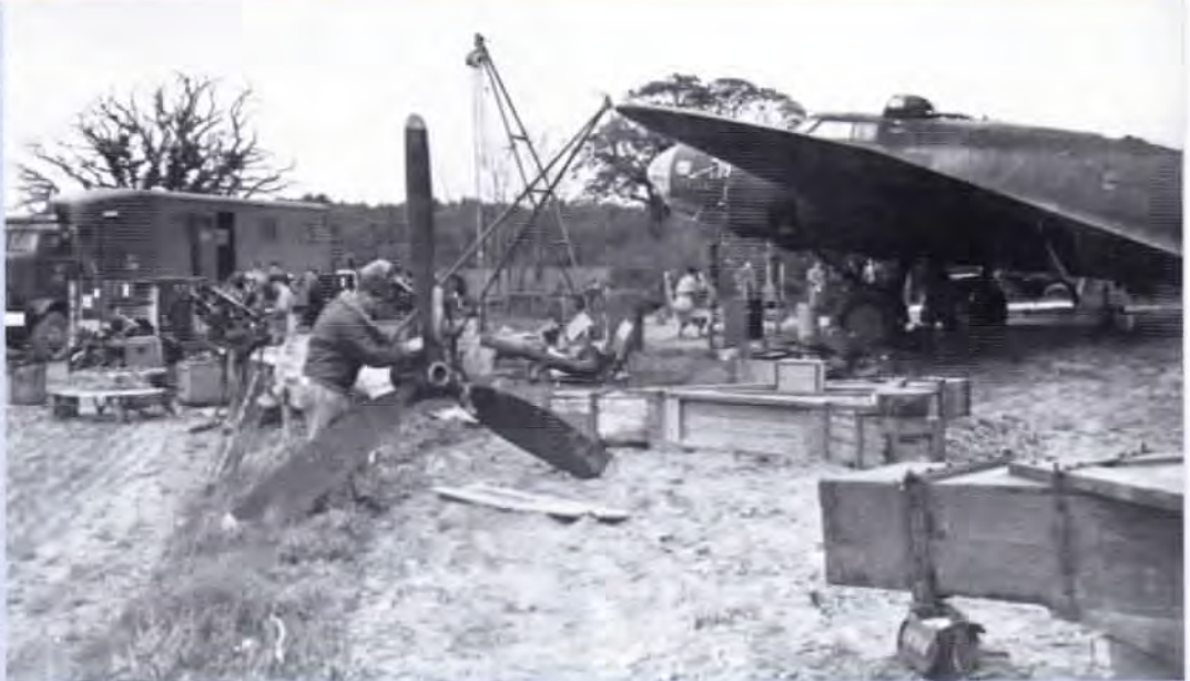
Replacing engines on B-17F Stella after an emergency landing.
