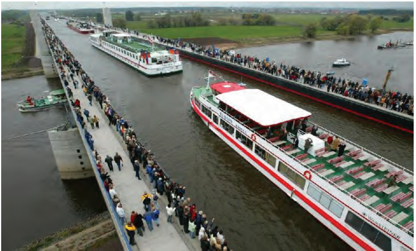
A water bridge crosses the river Elbe in the city of Magdeburg south of Berlin, joining the former East and West German countries. This feat of engineering took six years to build, cost 500 million Euros and measures 918 meters long. This photograph shows the bridge on its inauguration day. Farish Chandler, 491 st Bomb Group, states, "I thought six times to Magdeburg would finish their bridges, but at least it took them sixty years to build this one."
