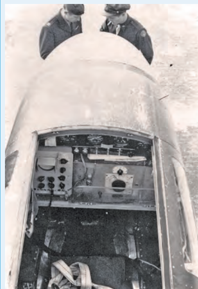
The cramped quarters of the Radar Observer in a 36th Bomb Squadron "Droop Snoot" P-38
