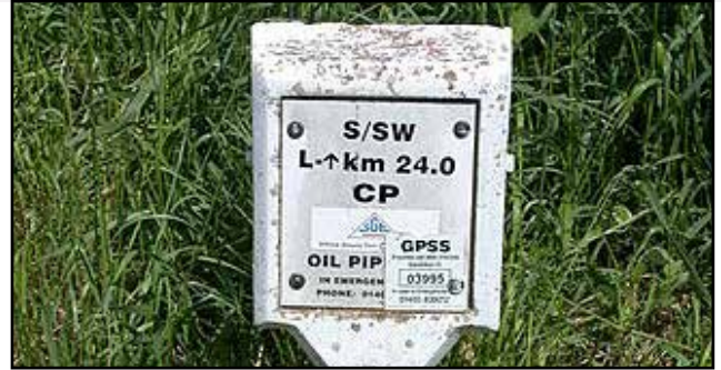
GPSS marker plate, near Heydon, Cambridgeshire. The marker text: S/SW shows marker is on the Sandy-Saffron Walden link; 24 kilometers (15 mi) is the distance from Sandy; up-arrow indicates that the normal flow is away from the observer looking at the notice. GPSS marker plate - geograph.org.uk - 833285
