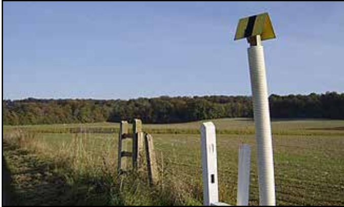
GPSS pre-World War II white marker, with post-World War II yellow/black post. The markers ensure that utility companies do not rupture the pipeline during construction projects. Oil pipeline marker - geograph.org.uk – 591698
